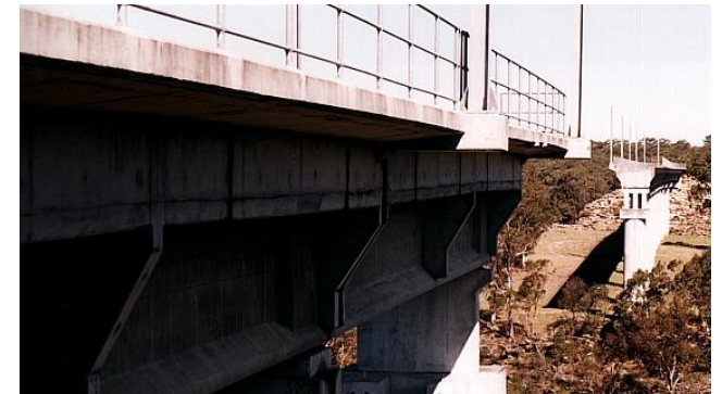
A BRIDGE TO NOWHERE? An unfinished bridge on the Maldon-Dombarton railway
